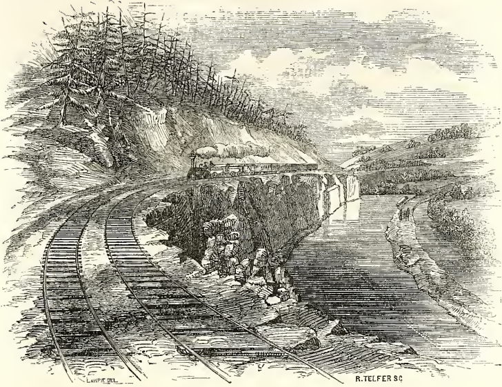
RAILROAD CURVATURE NEAR READING.
